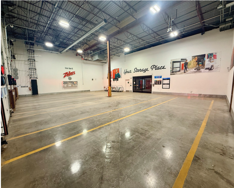
DRIVE-IN LOAD/UNLOAD AREA
