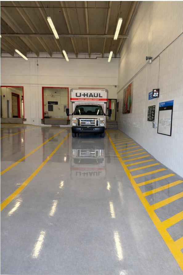
Drive-In Heated Load/Unload Area
