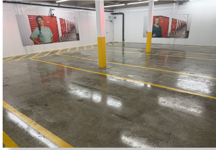
INDOOR LOADING AREA LOCATED ON BACK
